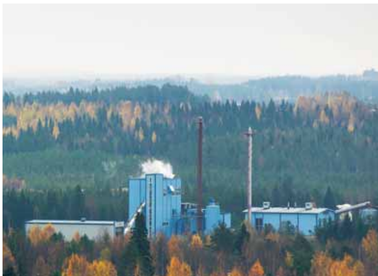
In the autumn of 2005, Vapo commissioned a unique production plant development, comprising a power and pellet plant in Ilomantsi.
