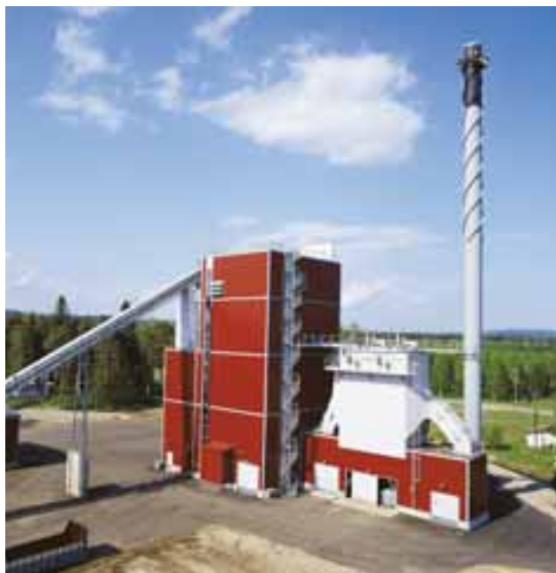
Vapo Energia's Lieksa power plant uses 4-6 truck loads of peat per day during winter.
