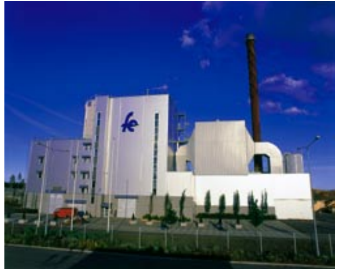
The power plant in Forssa utilises local biofuels: wood, peat and recycled fuel.
