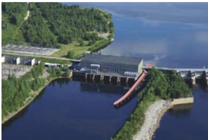
The three-year programme of implementing the Valajaskoski power plant's upgrading and raising of its power capacity was completed. At the same time, the river bed beneath the Valajaskoski Falls was cleaned out. As a result of these projects, the output of the plant, built in 1960, rose by 40 per cent.
